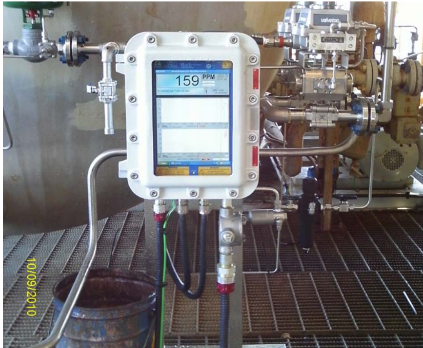
Figure 11: O&G Concentration of 159 PPM at the Skimmer Outlet.
