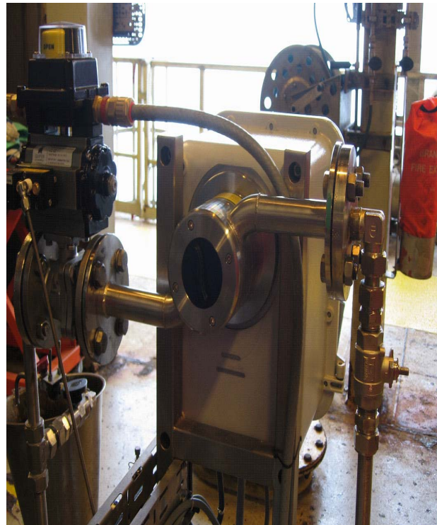
Advanced Sensors OIW-EX1000 monitor at Brage
