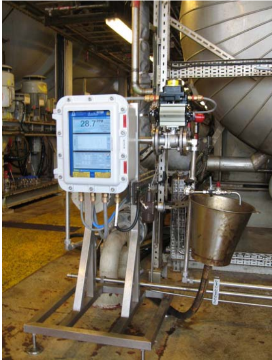
Advanced Sensors OIW-EX1000 monitor at Brage
